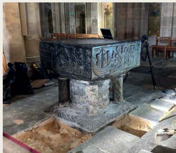
Conservation work on the Font commenced 2024 Photo: Winchester Cathedral
